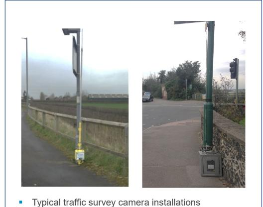
Camera mounted on top of pole (out of shot)
